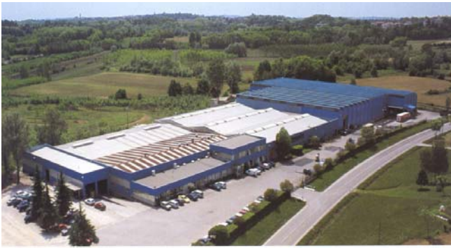
COMEFRI SpA factory at Magnano in Riviera (UD) Italy with 14.500 m 2 workshop. Production of radial fans for airconditioning and general ventilation.
